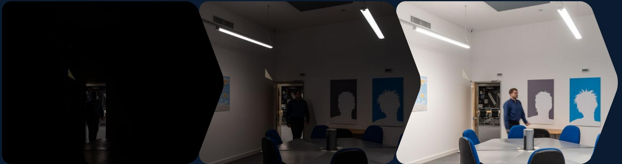
SmartScan Sensors are used to detect movement to turn the luminaires on. After a predetermined time of no movement the luminaires will turn off, saving energy. The sensors can be programmed for absence mode whereby the luminaires are not initially turned on automatically by movement, but manually by the user with a switch; the sensor will then monitor movement to turn the luminaires off automatically after a pre-determined time.
